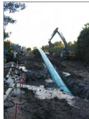
30" HDD Bore in Hillsborough, FL 2012
