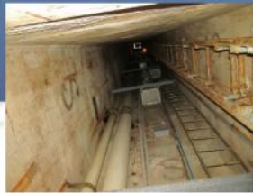
Vertical Shaft ~220ft
