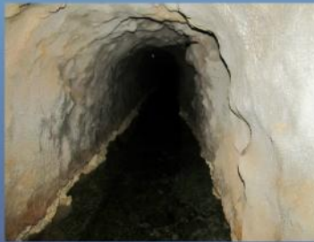
Southwest Infiltration Gallery ~200 ft long
