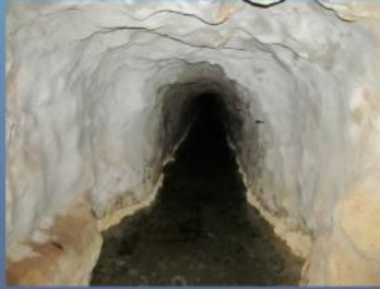
Southeast Infiltration Gallery ~200ft
