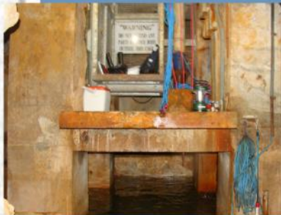
Platform and basin at the bottom of the shaft well
